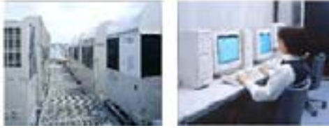
▲ Decentralized GHP Air Conditioning ▲ GHP Monitoring
